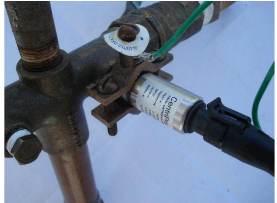
Figure 6: Attach Ground Clamp and Ground Wire
