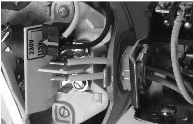
Figure 9: Voltage set to 115 volts, Plug Type
