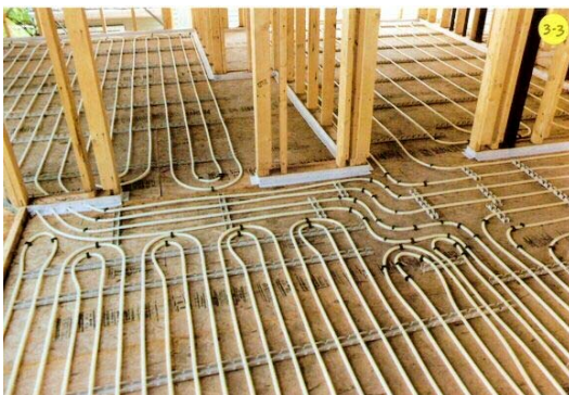
Figure 2: Typical tubing layout on a residential radiant heating installation. [ref: Photograph by John Blais for TOH Magazine]
