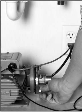
3. Attach shut-off flanges to pump.
