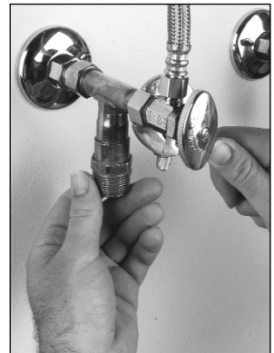
2. Install tees and attach angle stops.
